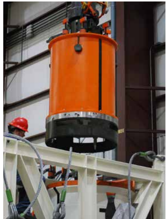
Installation of HIPPS Control Pod
