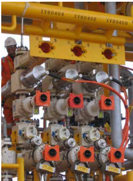
HIPPS Pressure Sensor Header for production manifold-based application with multiple trees
